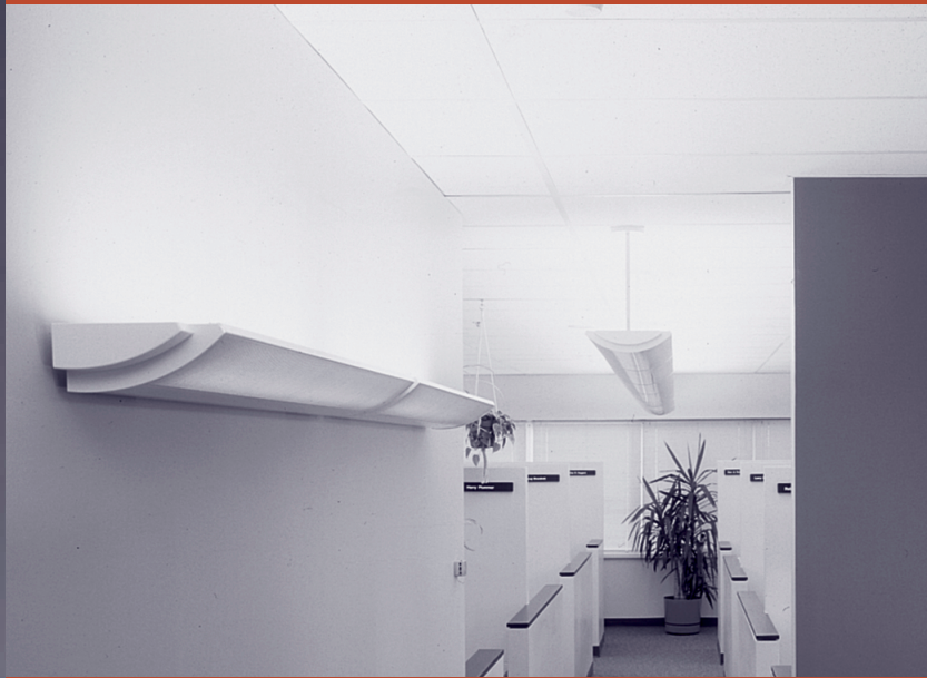
Swanson Rink Mechanical & Electrical Consulting Engineers, Denver, CO Matt Slater, Photography
